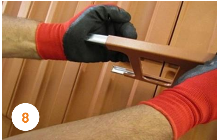
8 Use the two joiner to connect the grids to avoid the further deflections!
