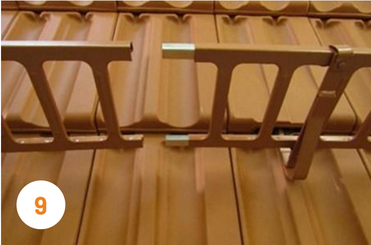
Place the joiners to the rail by hand.
