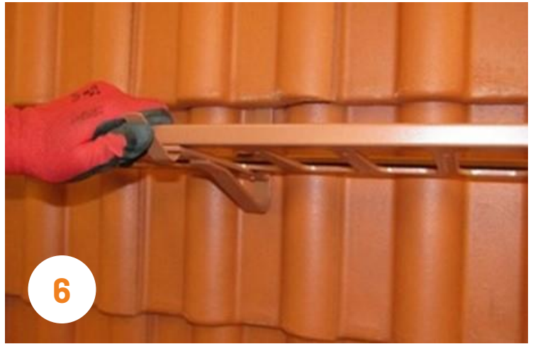
6 Place the grid to the rail! The overhang of the grid has to be lower than the \frac{1}{3} part of the support distance!
