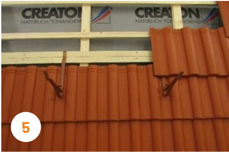
5 Finish the tile cover and place base tiles above the supports!
