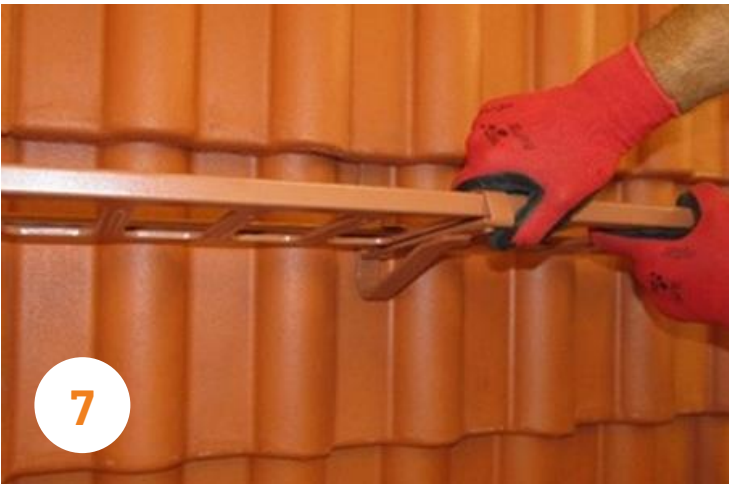
7 Blend the upper fixing plate by hand to fix the grid!
