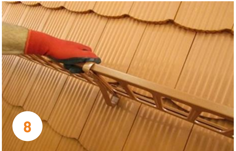
Blend the upper fixing plate by hand to fix the grid!!
