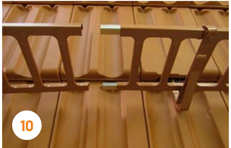
Place the joiners to the rail by hand.
