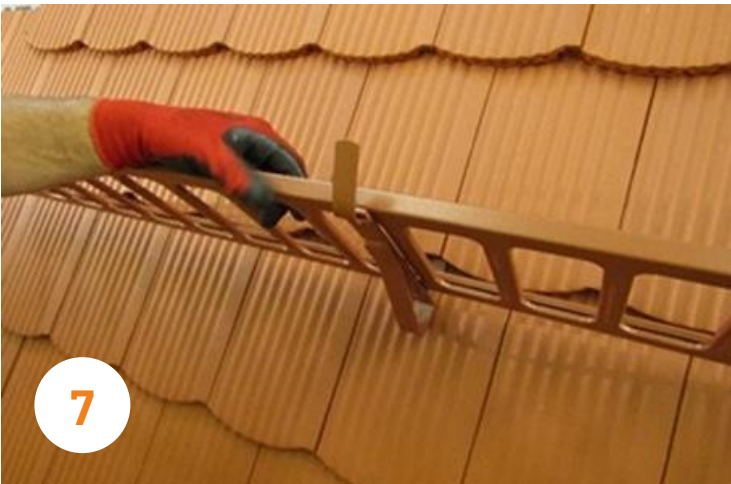
Place the grid to the rail! The overhang of the grid has to be lower than the \frac{1}{3} part of the support distance!
