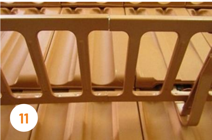
The connection does not require additional fixing!
