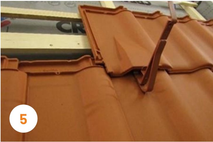
5 Finish the tile cover and use the ventilation tiles above the snow guard grid supports!
