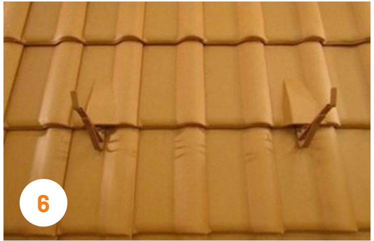
6 For some tile model you have to broke out one or more support in the ventilation tiles! You can find further information about this in the end of this guide!
