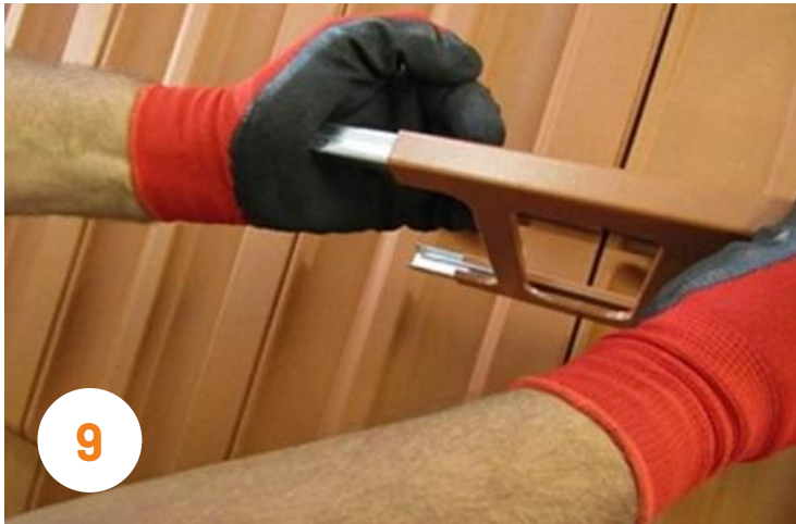
Use the two joiner to connect the grids to avoid the further deflections!
