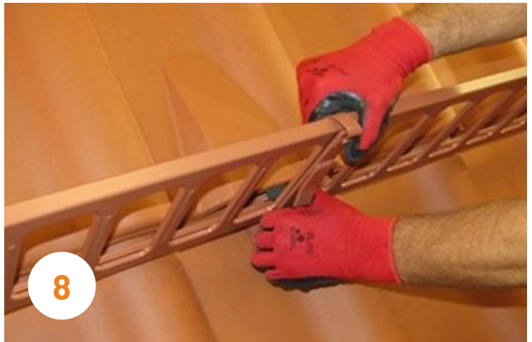
8 Blend the upper fixing plate by hand to fix the grid!!
