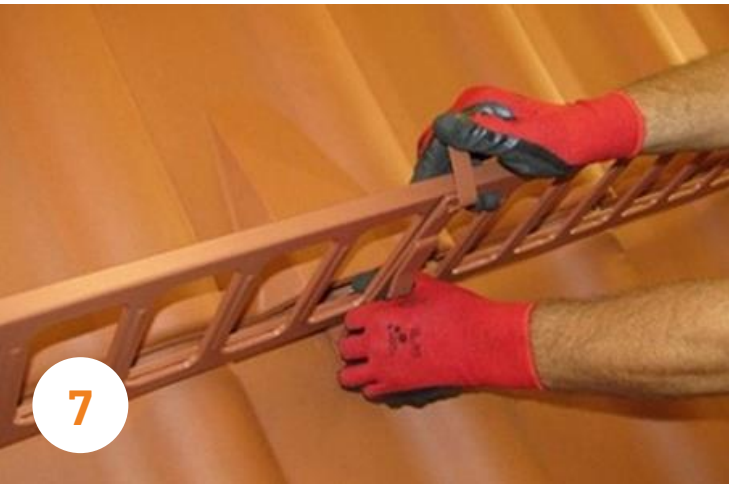
7 Place the grid to the rail! The overhang of the grid has to be lower than the \frac{1}{3} part of the support distance!
