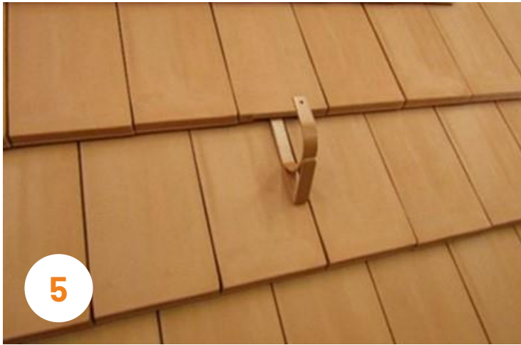
Finish the tile cover and use the ventilation tiles above the safety hook!
