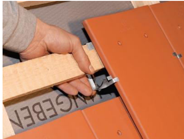
Mount-on stormclip for plain tiles
